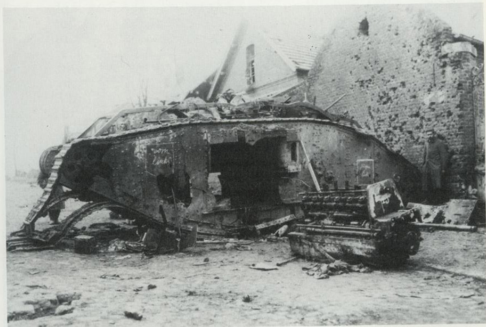
With the Mark IV, of which more than 1000 were produced in Britain, the "tank" appeared on the battlefields of 1917-18 as a new weapon. The first tanks could be stopped only by a direct artillery hit, as has happened here.
